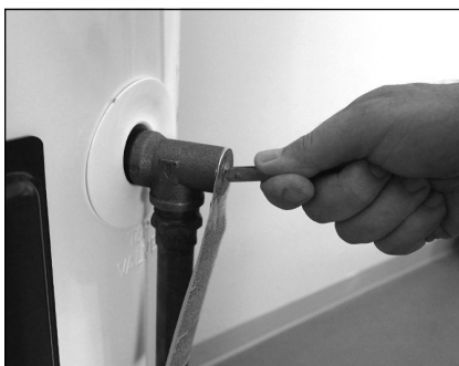
Figure 38 - T&P Relief Valve
