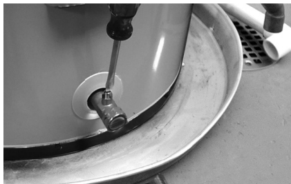
Figure 10 - Draining the old water heater.
