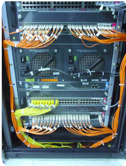
Figure 1 - Patch Panel - Examples
