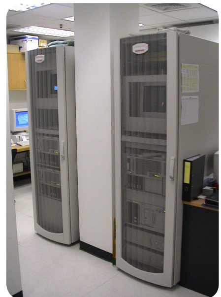
Figure 7 - Server Racks - Example
